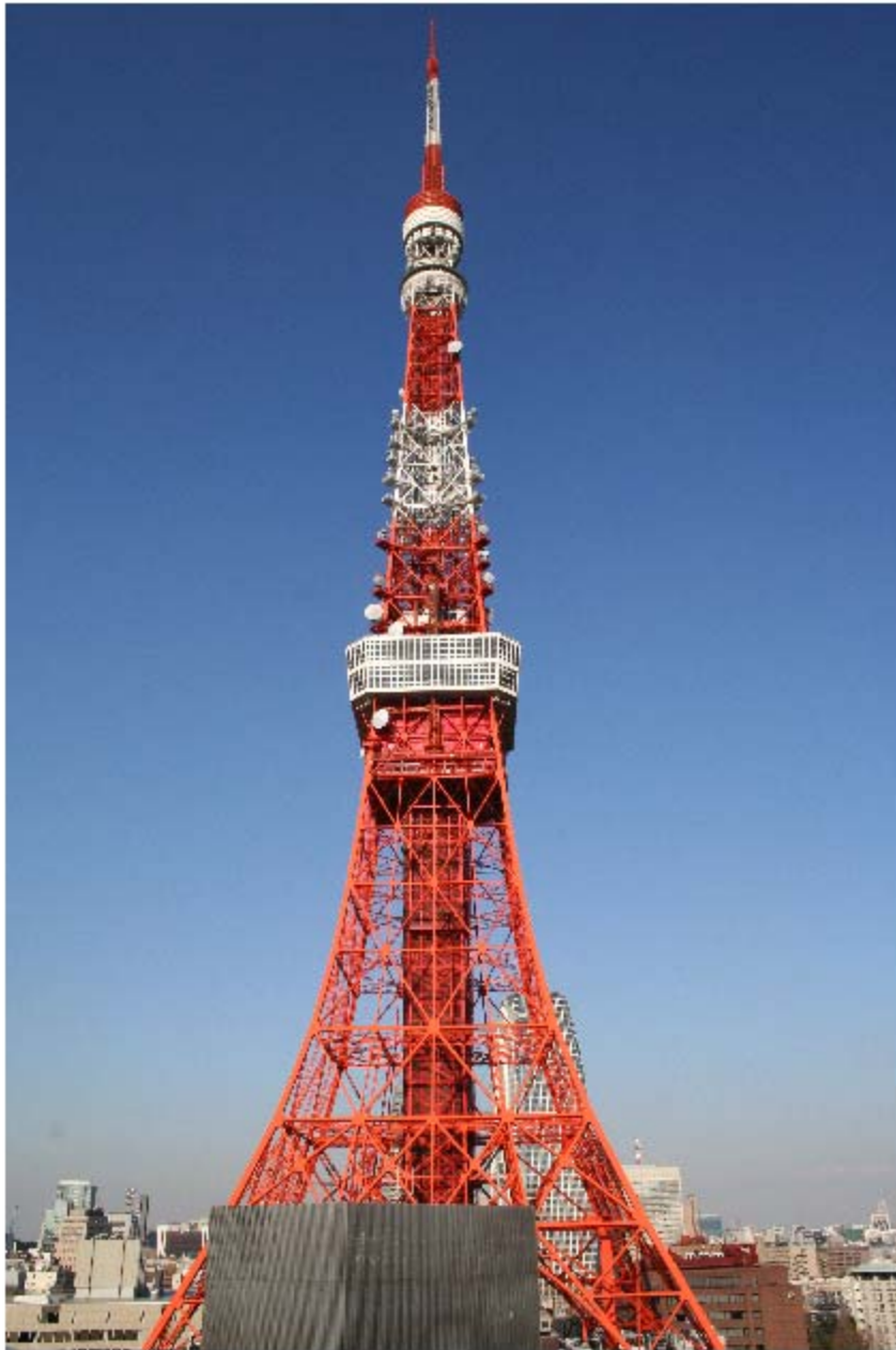
World's Tallest Communications Tower - Japan
